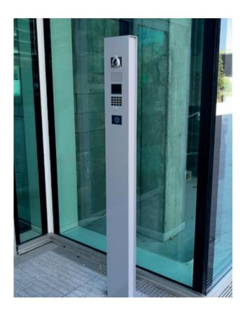
The entire intercom system has been connected to the Siemens Siveillance BMS system for management and diagnostics.
