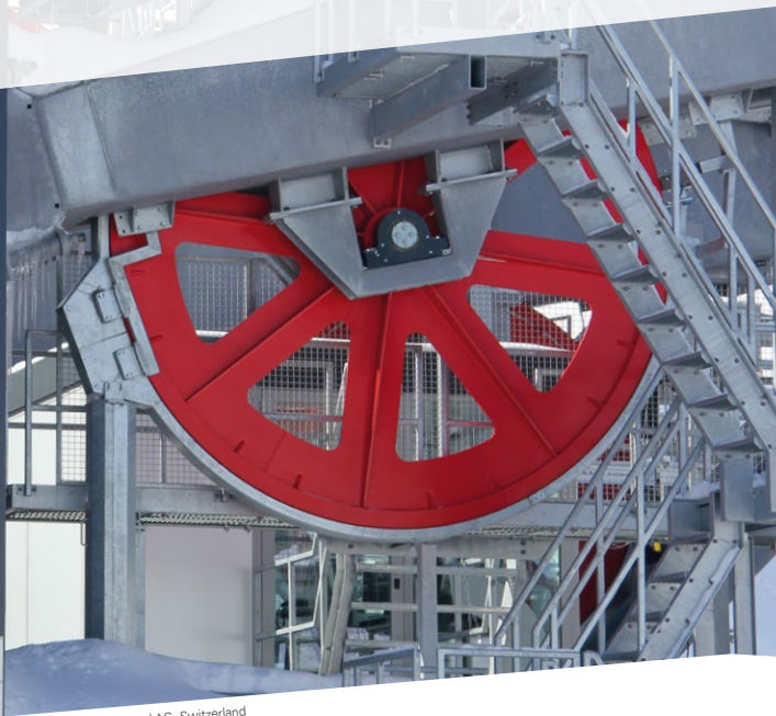
Photos: Commend AG, Switzerland
